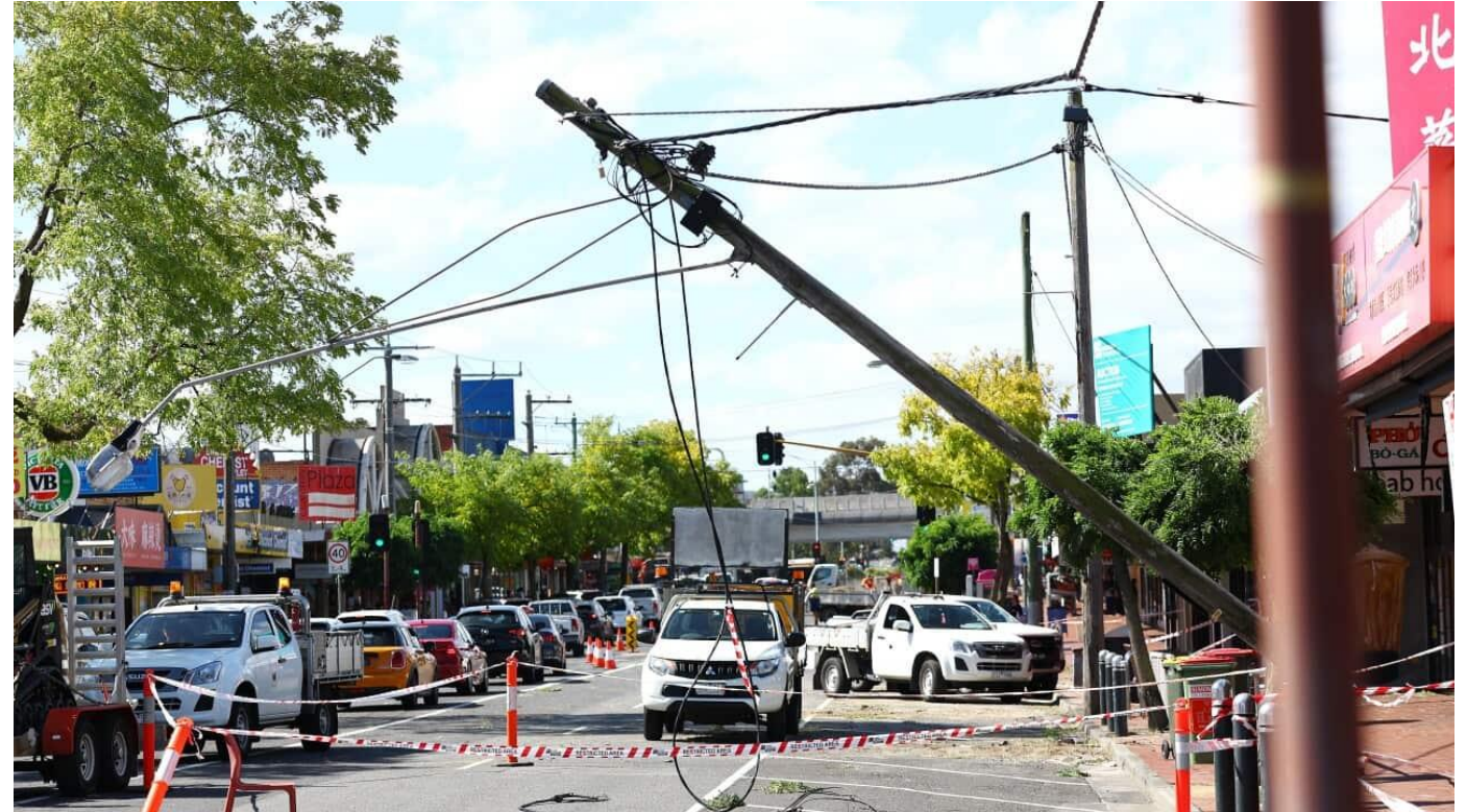
Storm damage 13 Feb 2024
